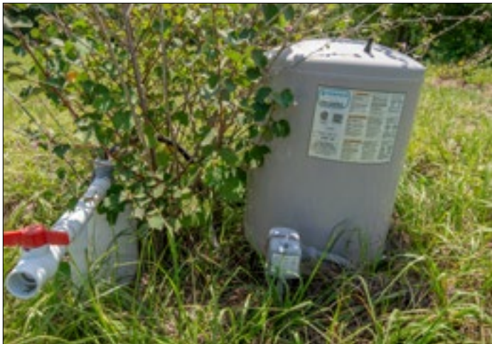
New 5-inch well with 1.5 HP submersible pump
