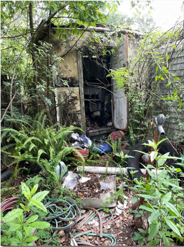
Look south at soil boring B30 location in front of a shed 15 feet west of dilapidated Shed 2.
