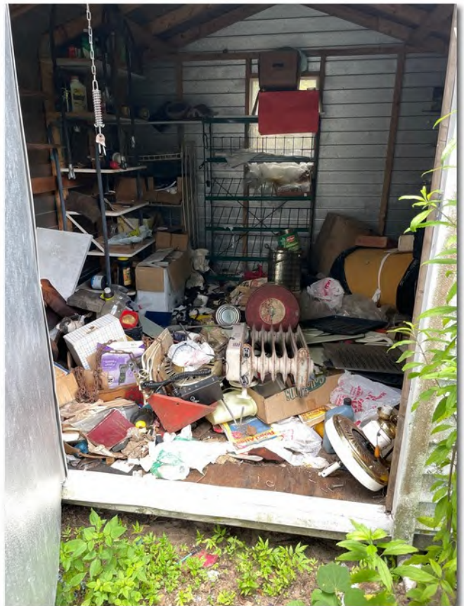
Inside of a shed 20 feet west of dilapidated Shed 2
