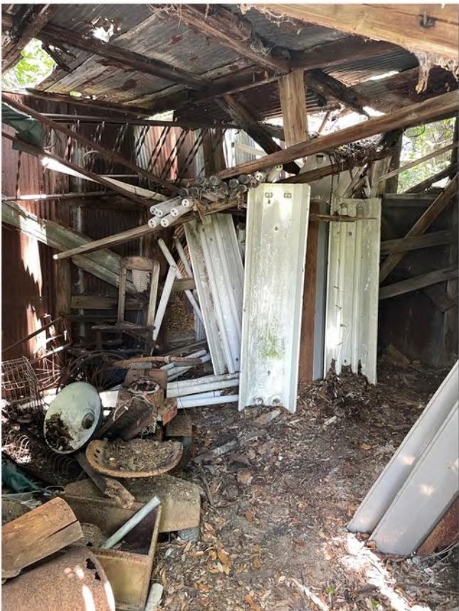
Fluorescent tube storage location at North Pen soil sample location
