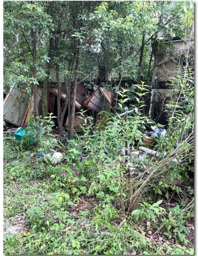
Looking southeast at dilapidated Shed 2
